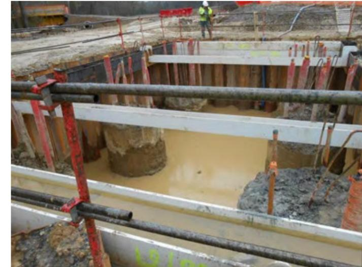
FIGURE 355 : EXEMPLE DE BATARDEAUX AU NIVEAU DES PILES (BATARDEAU EN ZONE INONDABLE) [ARTELIA]
