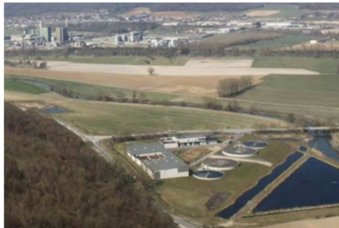
FIGURE 61 : STATION D'EPURATION DE LERY [ARTELIA©, 2013]
